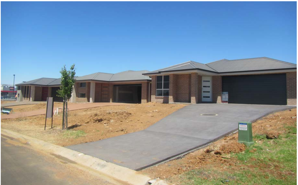
Photograph 7: Compact single residential housing under construction located to the north of the subject site
