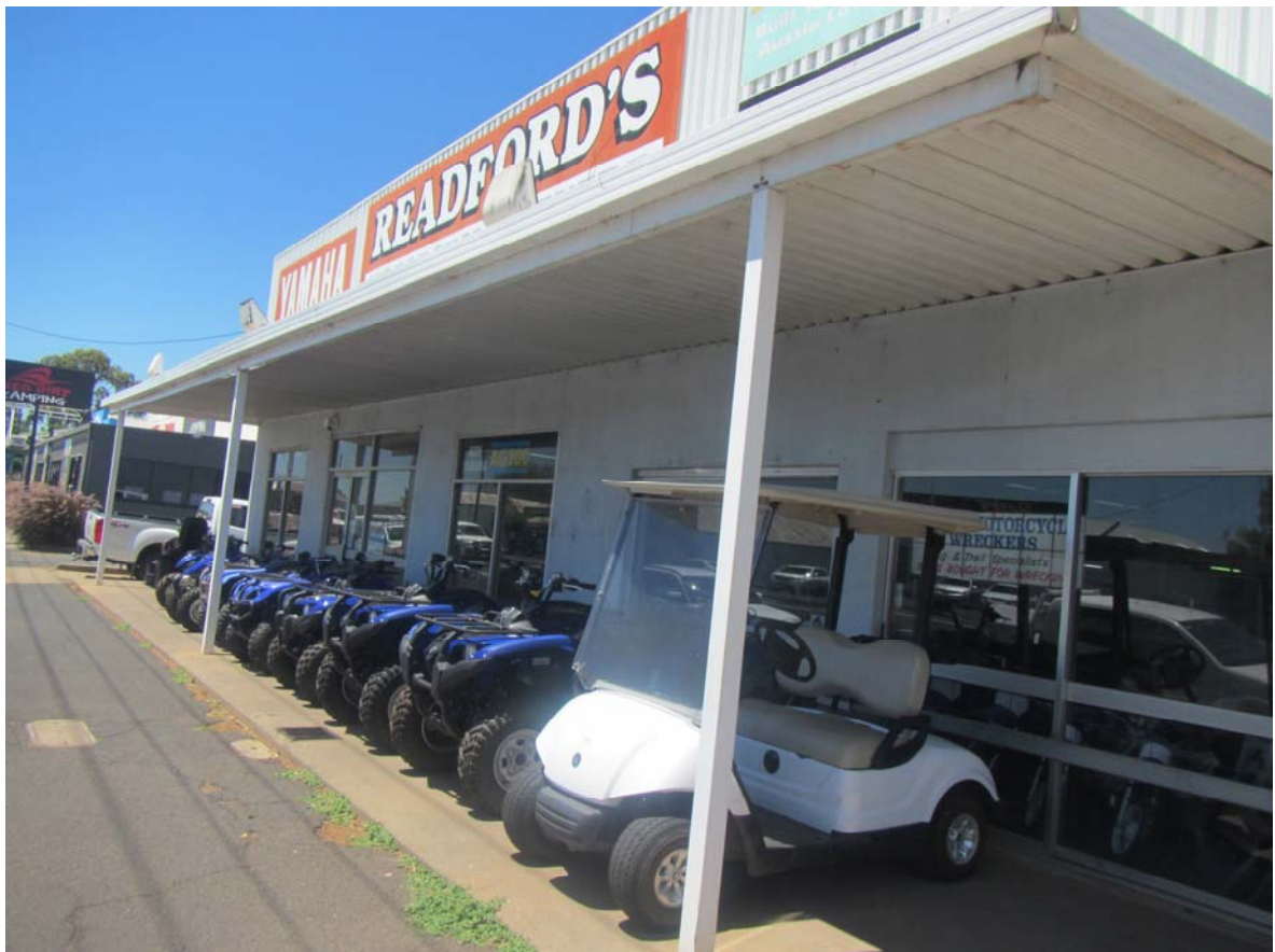
Photograph 8: Automotive uses prevail within the B6 zone on Mitchell Highway
