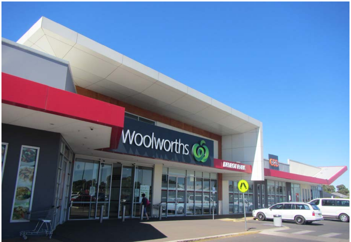
Photograph 1: Existing Development of the site
